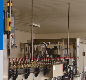
Automation / Process Control
